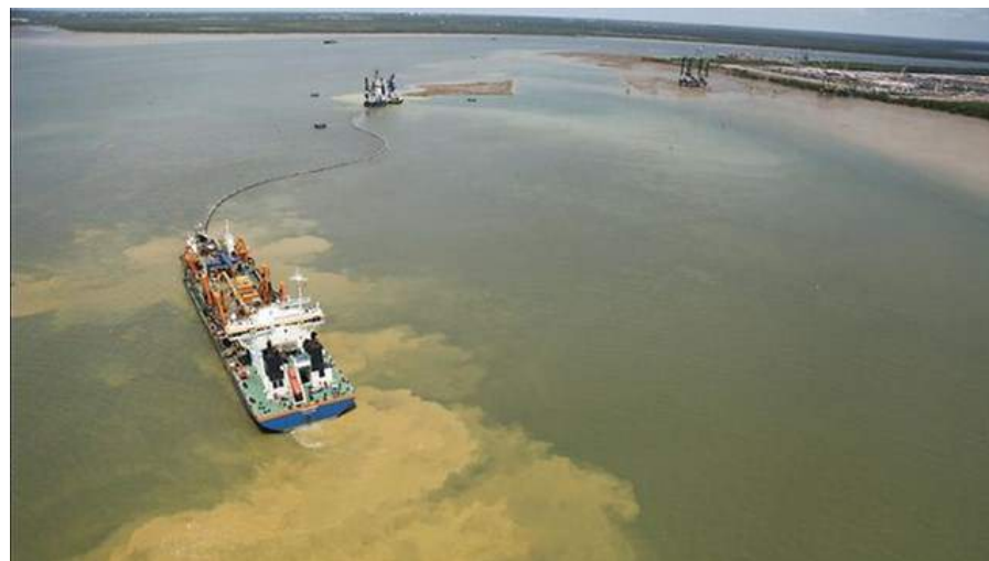
Photo 7.1 ► Example of a Dredger at Work has Caused Turbidity Plume Source: http://resources0.news.com.au/
